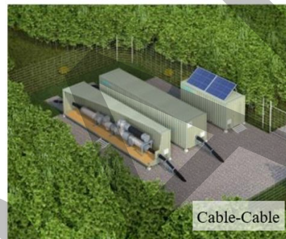
Figure 3 – Typical cable-cable intermediate transition station
