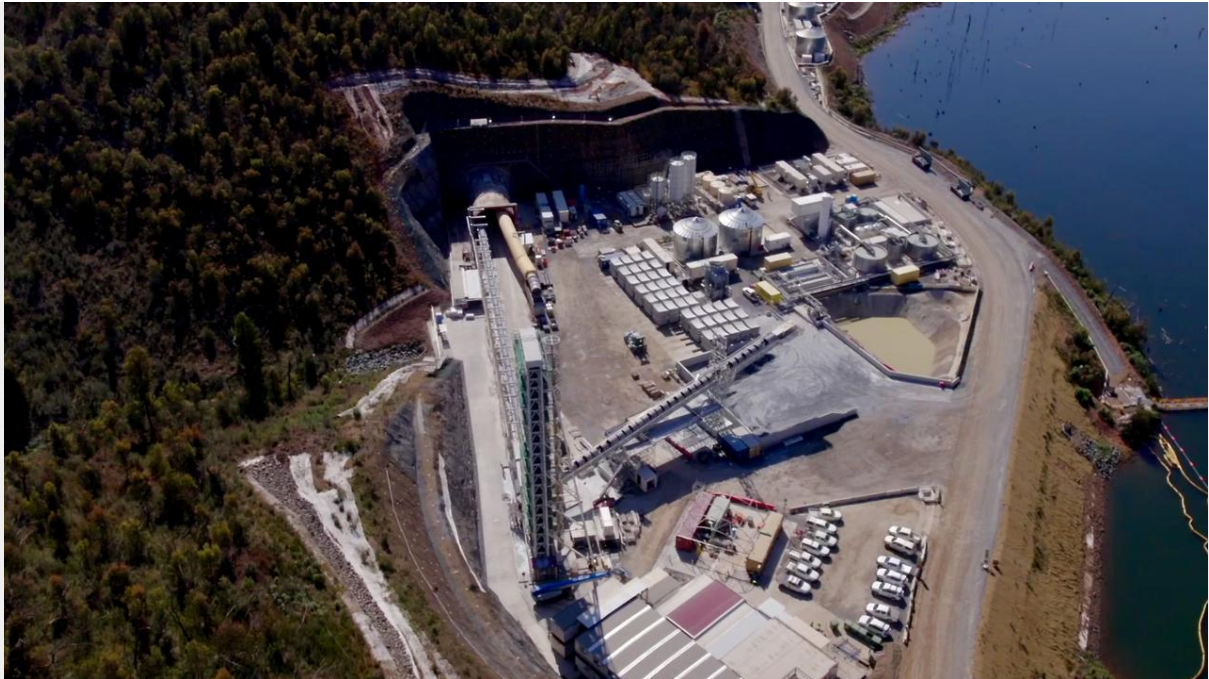
The Snowy Hydro 2.0 project.
