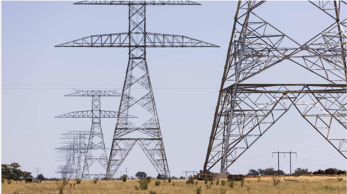
Transgrid transmission lines running over rural properties. Picture: Ash Smith
