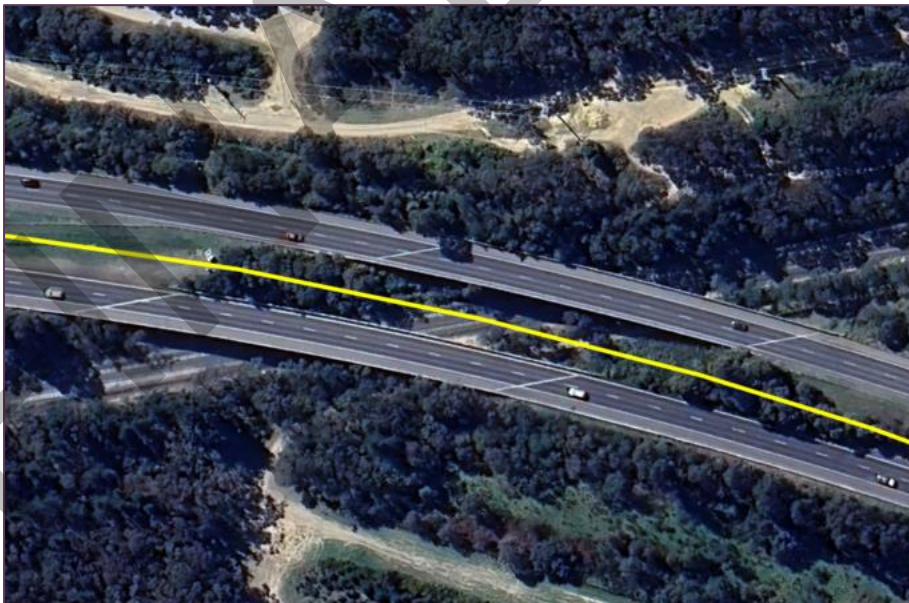
Figure 43 - Example of a crossing of a well vegetation road/rail overpass (Source: Google Earth).
