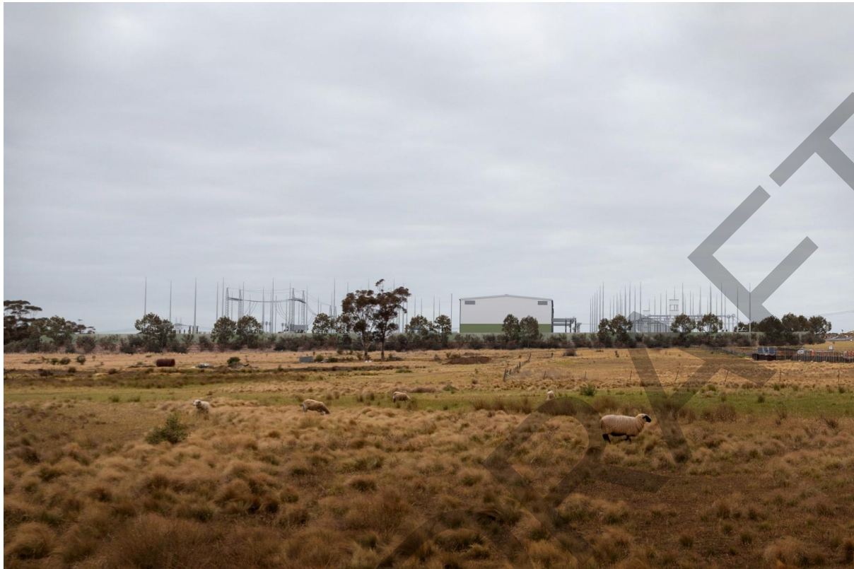
Figure 79 - Photo simulation view from Holden Road to the Project with establishing vegetation at 5-7 years post construction.
